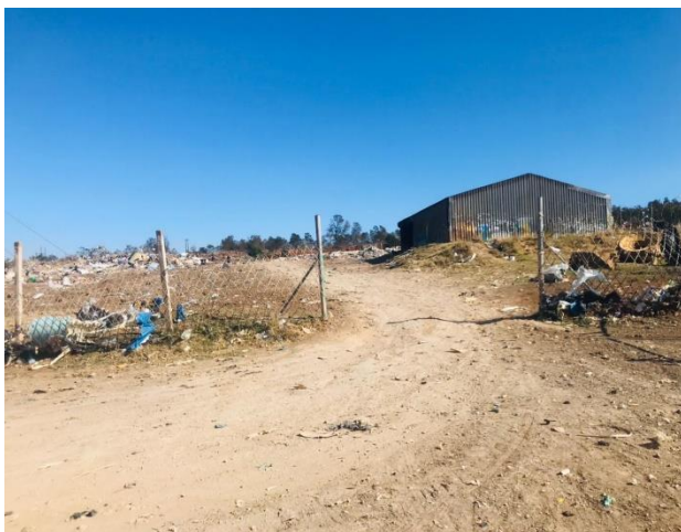
Figure 9: Material Recovery Facility in Stutterheim
